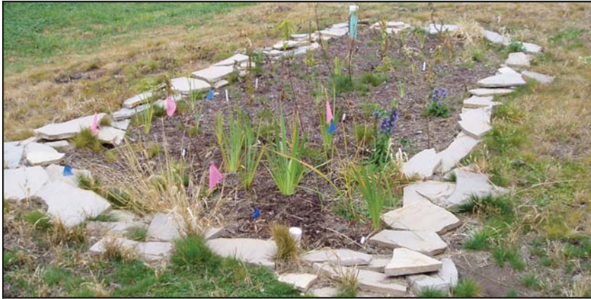
The second polishing wetland, installed after the Dyno2 wetland system. This cell discharges to the rain garden.
